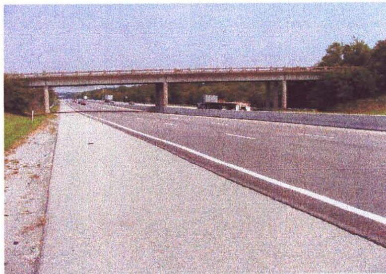
LOOKING AHEAD ON ROUTE (94-I65-0.85 UP.)
