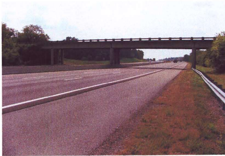
LOOKING BACK ON ROUTE (94-I65-0.85 UP. )
